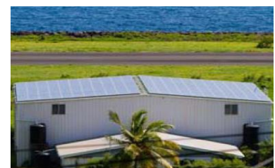
Hanger at Bequia Airport with solar panels installed on the roof
